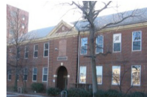
Building 661 awaits its transformation
